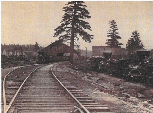
The Truckee Depot. Two additional locomotives were hauled and skidded to Truckee
